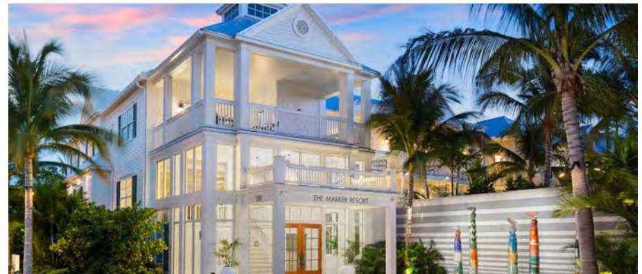
THE MARKER KEY WEST HARBOR RESORT, KEY WEST, FLORIDA
